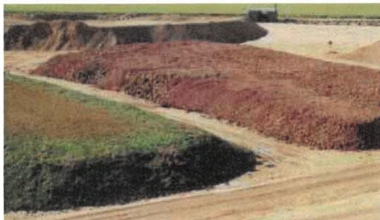
Clearly defined stockpiling of different soil materials
