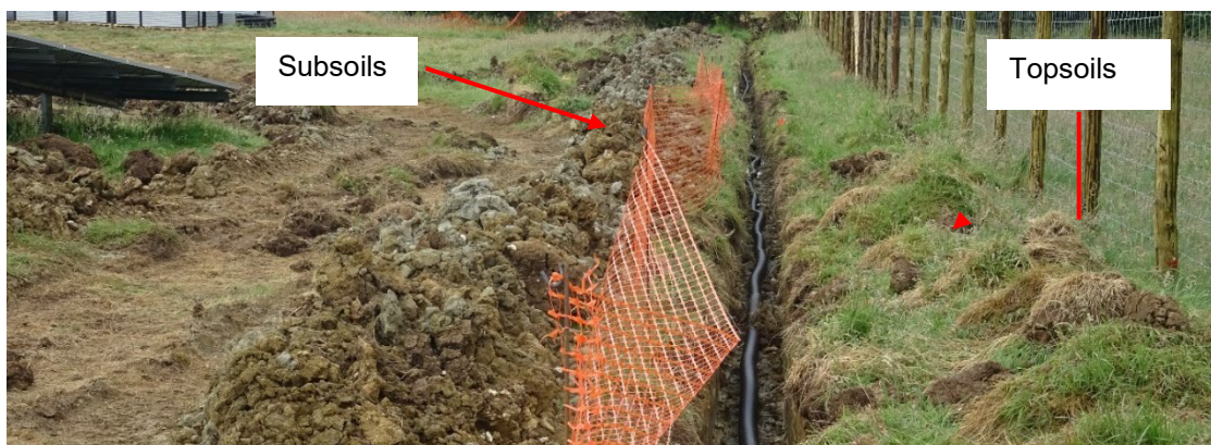
Insert 42: Subsoils Dug out of the Trench
