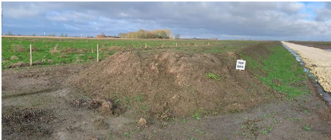
Insert 8: Temporary Topsoil Storage (January 2023)
