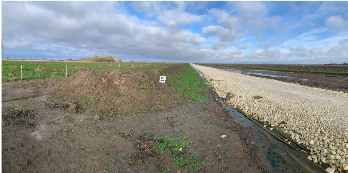
Insert 13: Temporary Topsoil Storage (January 2023)
