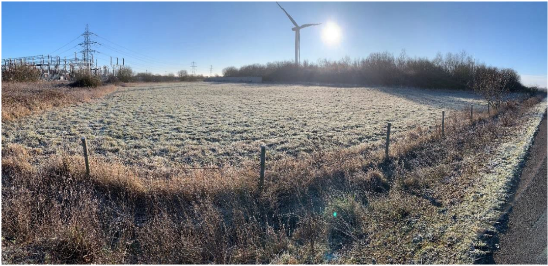
Position 19: Small grassland area at the substation
